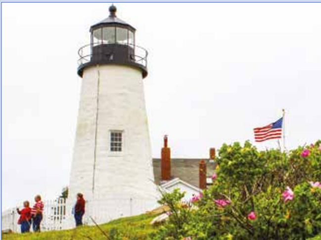
The lighthouse at Pemaquid Point
