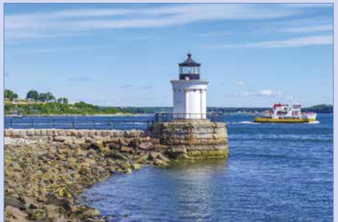
The Portland Breakwater light
