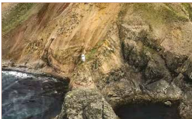
The leaning lighthouse before any secure measures were in place
