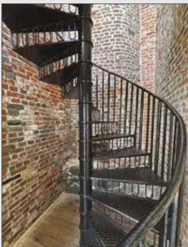
The original spiral staircase
