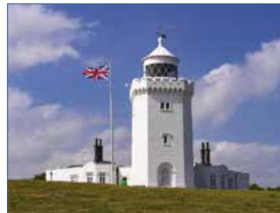
South Foreland lighthouse
