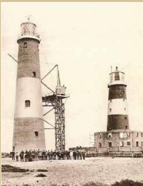
Shortly after the 4th lighthouse at Dungeness was completed in 1910, the 3rd lighthouse (right) was demolished, leaving just the 1843 Round House base.
