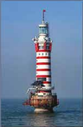
Dagu light, China (1978). No room for everything inside? Just bolt it to the outside.
