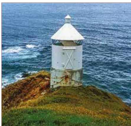
Gjögurtá standing erect in 2001
