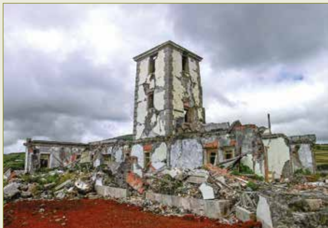
The Ribeirinha light after the 1998 Azores earthquake. Photo from Wikiwand
